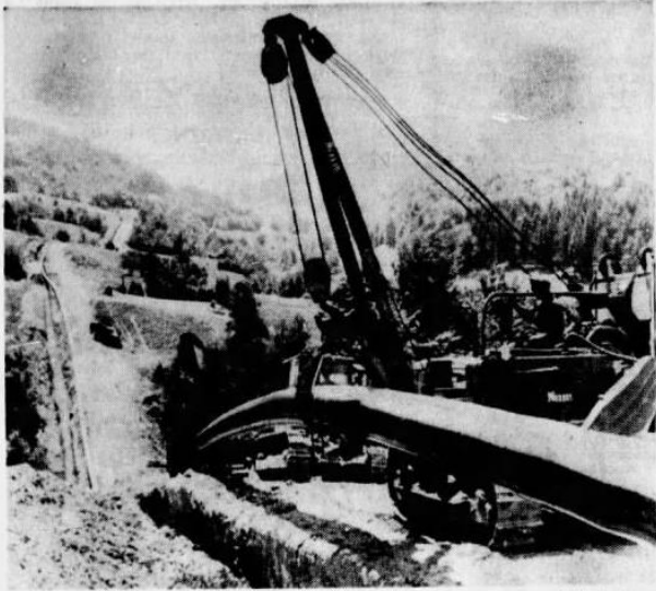
AP Wirephotos A Western embargo on Russia's efforts to purchase urgently needed "big inch" pipe to complete construction of a giant system of oil and gas lines is seriously delaying construction. This is a section of Russia's oil pipeline in the Carpathian mountains. The pipeline is called "Druzhba," or "Friendship."
