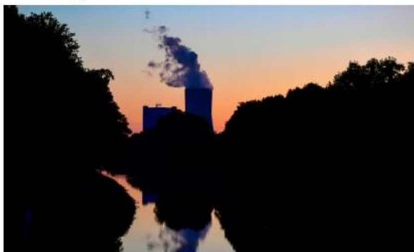
▲ The cooling tower of a coal-fired power plant in Datteln, Germany. Photograph: Ina Fassbender/AFP/Getty Images
