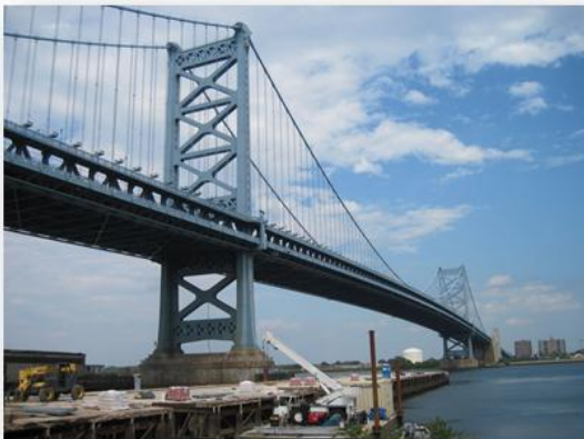
Ben Franklin Bridge in Philadelphia Opened January 6, 1922 The largest single span suspension bridge in the world, at 1.8 miles
